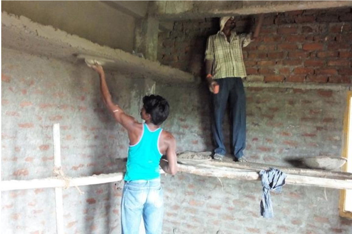
With water the workers are busy building walls
