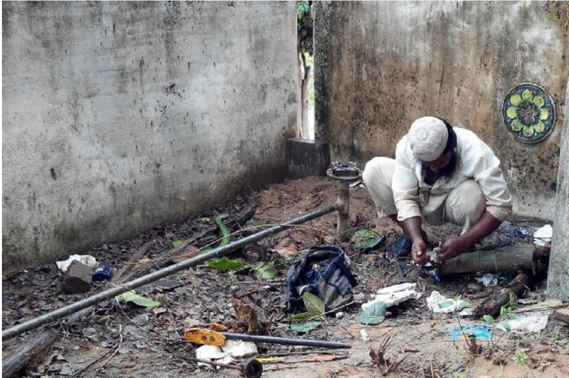
The water supply getting upgraded
