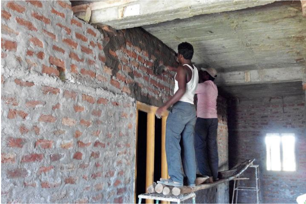
Busy workers preparing to stucco the wall
