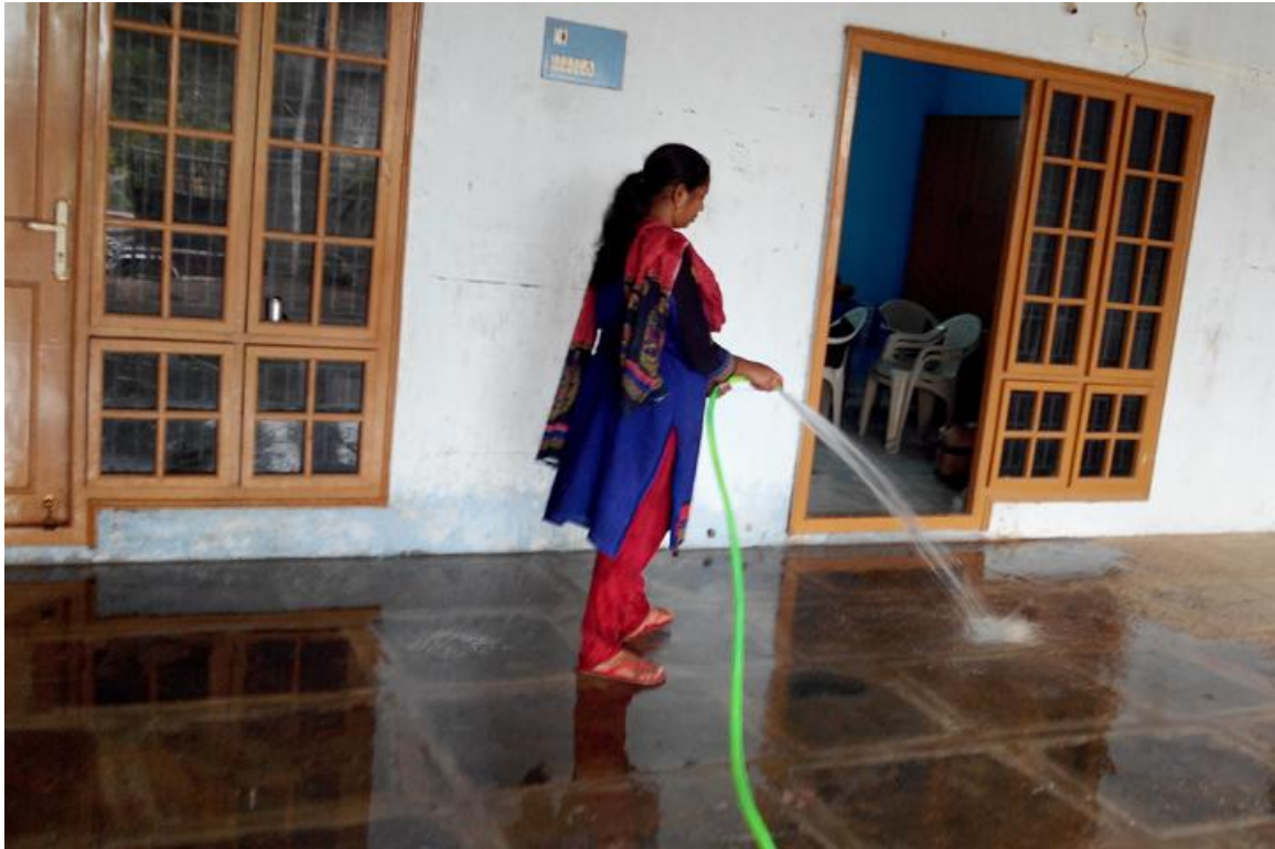
An almost completed area with more to come
